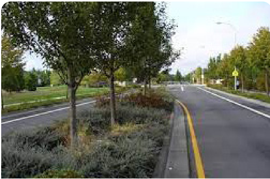
Traffic Calming median with low maintenance vegetation
