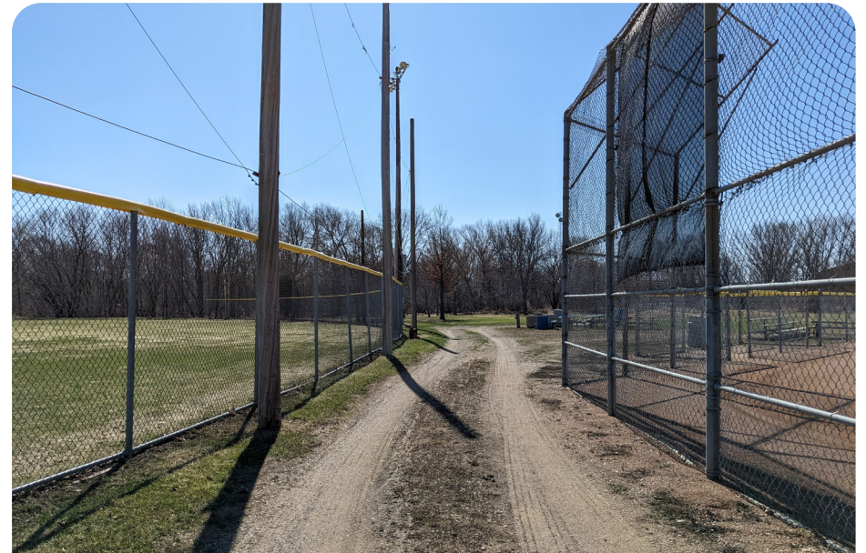
Gravel pathways are located between and around the ballfields.
