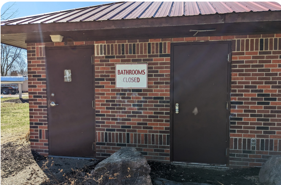
Restroom building east of the Vermillion River
