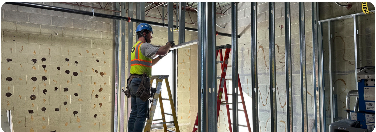
Stacey's office and the new reception area are being framed in.
