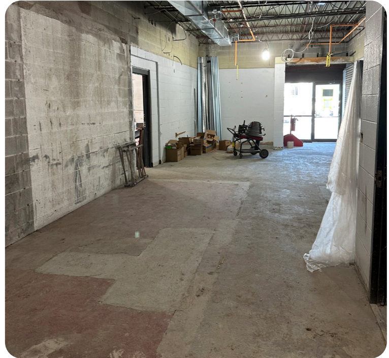
The jails cells and plumbing have been removed.
